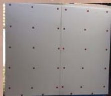
Fixing 50mm polystyrene boards & fastened to wall studs.
