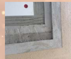
Complete stages of Fireshield Render System
